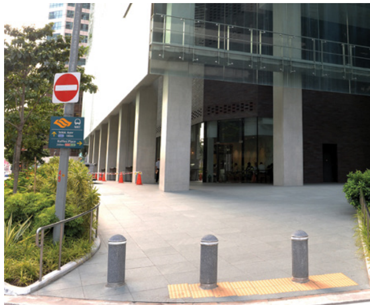
This raised development in Robinson Road is an example of a local measure to reduce flood risks in building developments.
